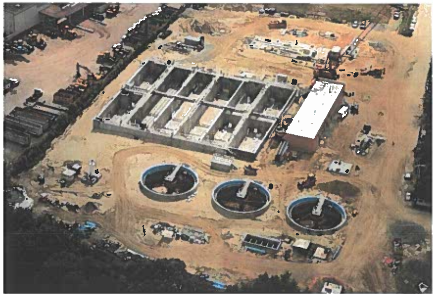
Maple Avenue Wastewater Treatment Plant during construction.
