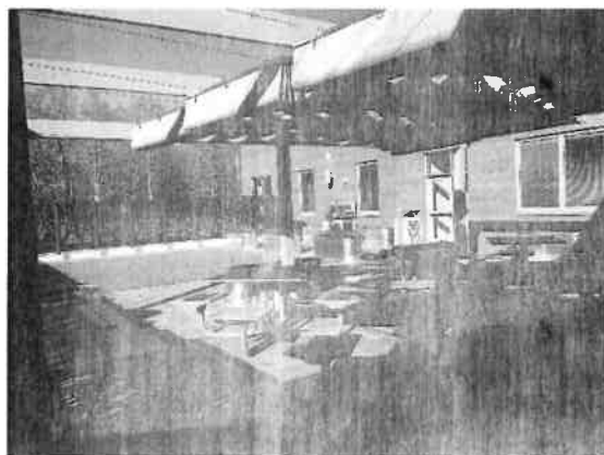
Roof Terrace- Construction Progress Photo
