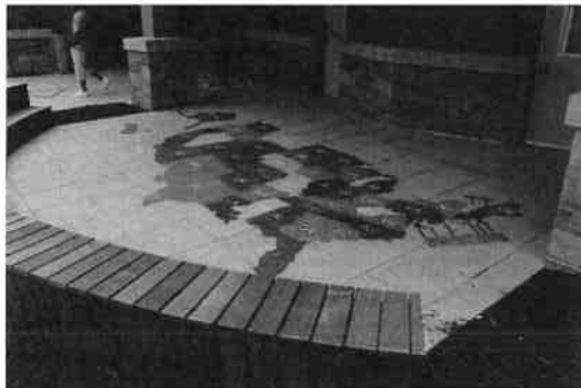
Main Courtyard- Construction Progress Photos
