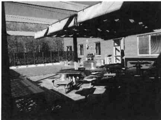
Roof Terrace- Construction Progress Photo
