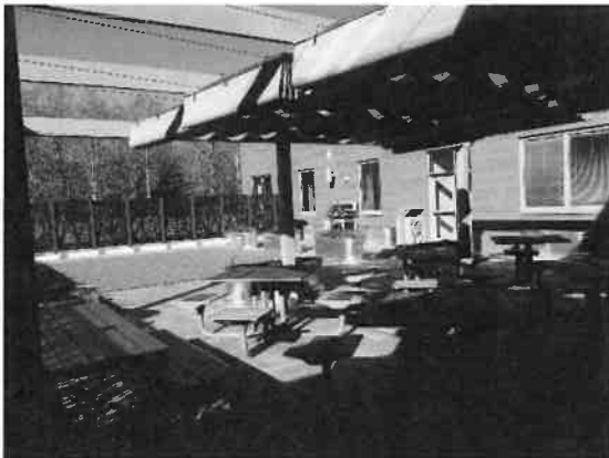
Roof Terrace- Construction Progress Photo
